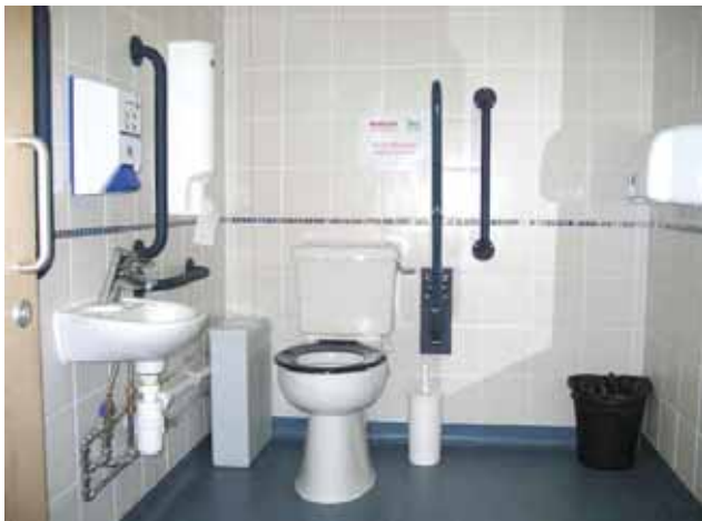
Good visual contrast between WC pan and seat. Note also the contrasting colour of the grab-rails from the wall
